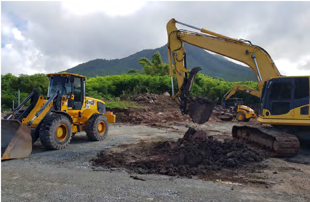
Figure 7.6: View from Project Site Looking East
